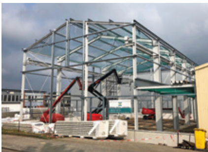
The new hall increases production capacity and creates space for the construction of large machines that are completely assembled and tested in Roetgen. © Hellweg Maschinenbau GmbH & Co. KG, Roetgen
