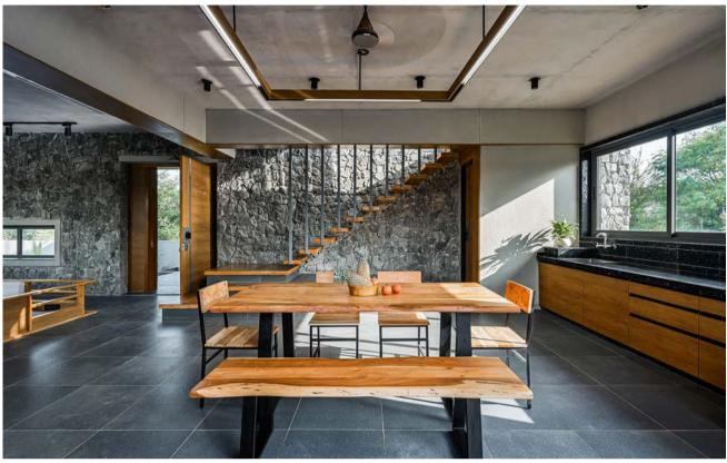
"The house is constructed using a combined structural system; with load-bearing stone walls and an external frame structure in steel with a butterfly roof. This binary relationship between the two materials creates an interesting experience."
